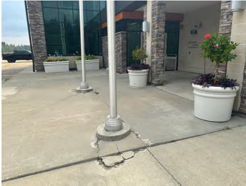
Figure A2: Spalling around Second Pole
