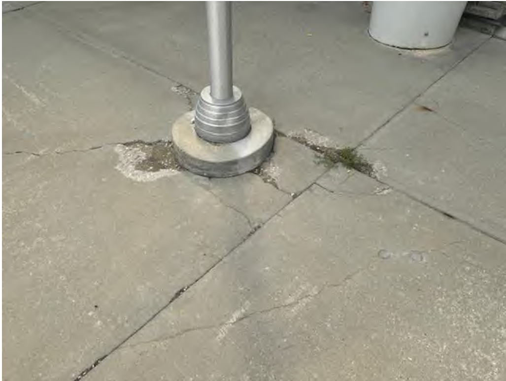
Figure A6: Cracks at the Bottom of the First Pole
