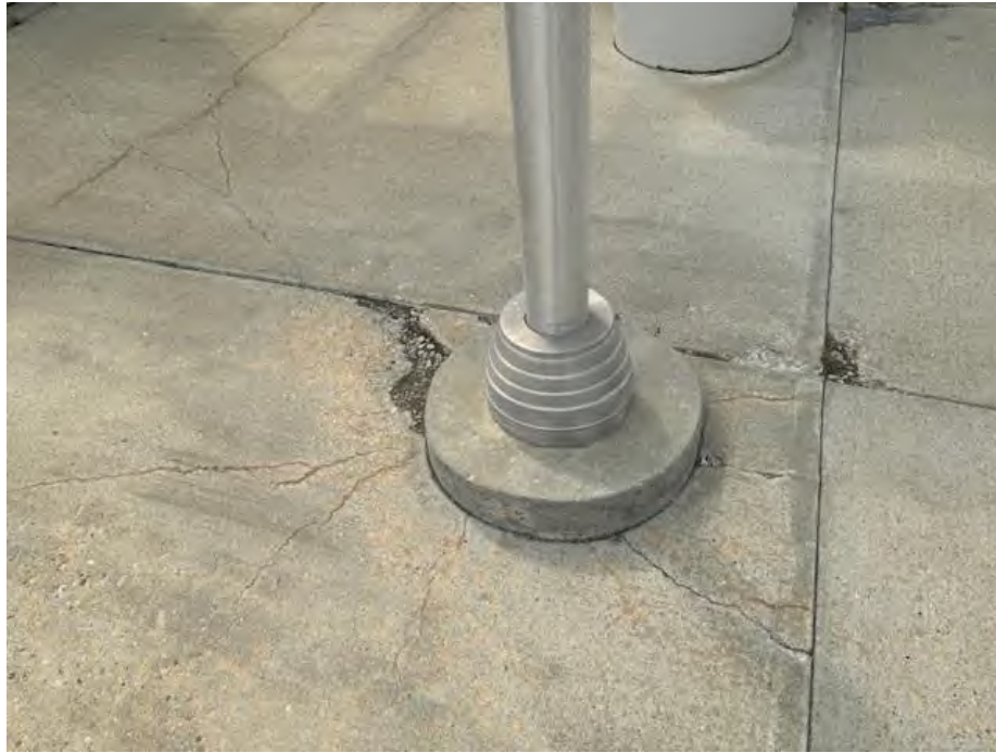
Figure A8: Cracks and Spalling around the Third Pole
