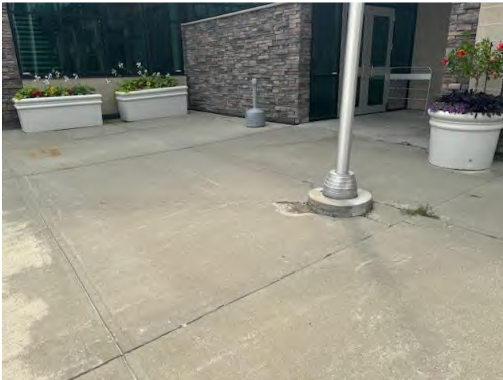
Figure A5: Spalling around the First Pole
