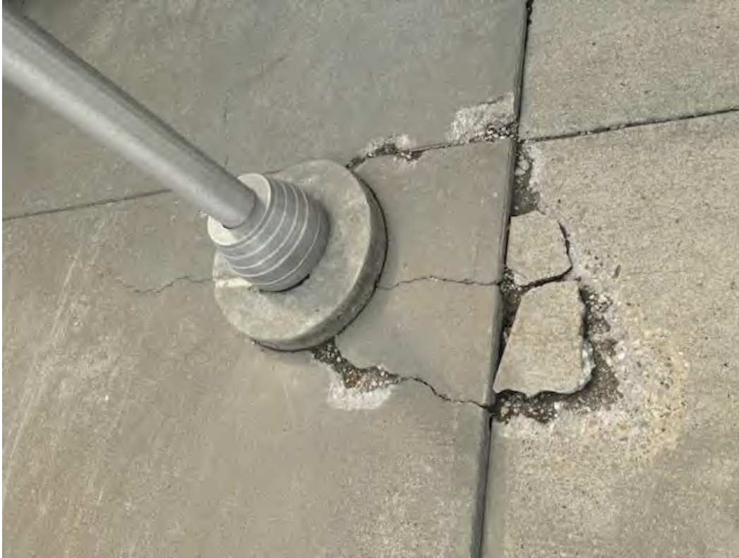
Figure A4: Cracks at the bottom of the Second Pole
