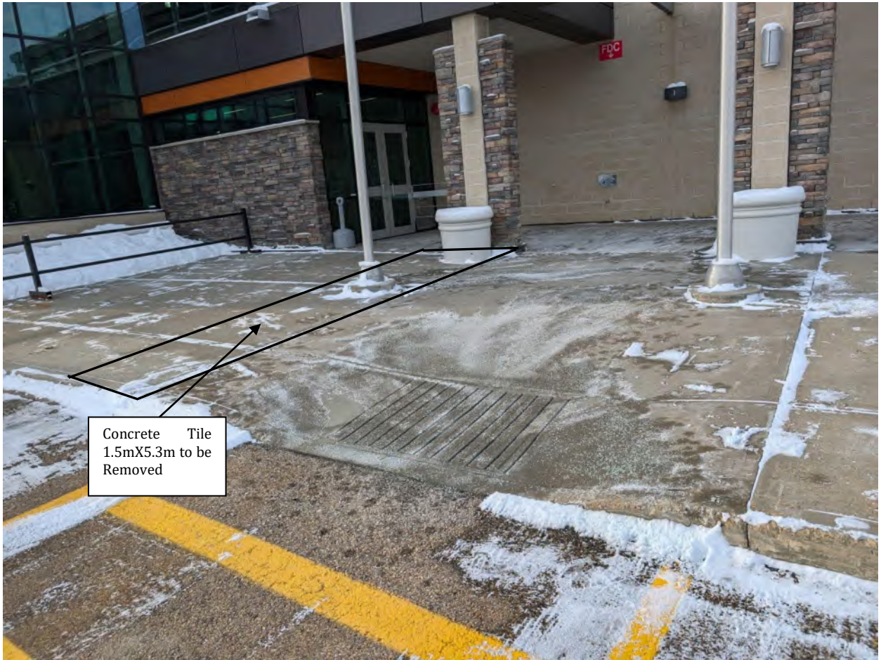
Figure A12: Area to be Saw Cut around P1
